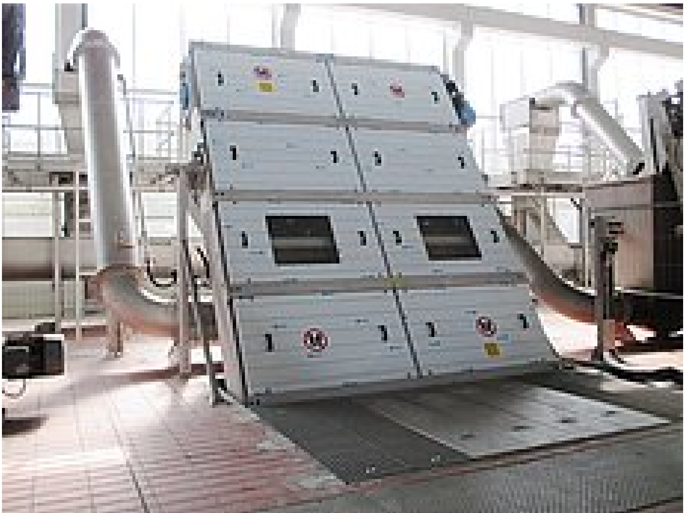
One of the broad HUBER Multi-Rake Bar Screen RakeMax® units with 8 mm bar spacing used as coarse screens
