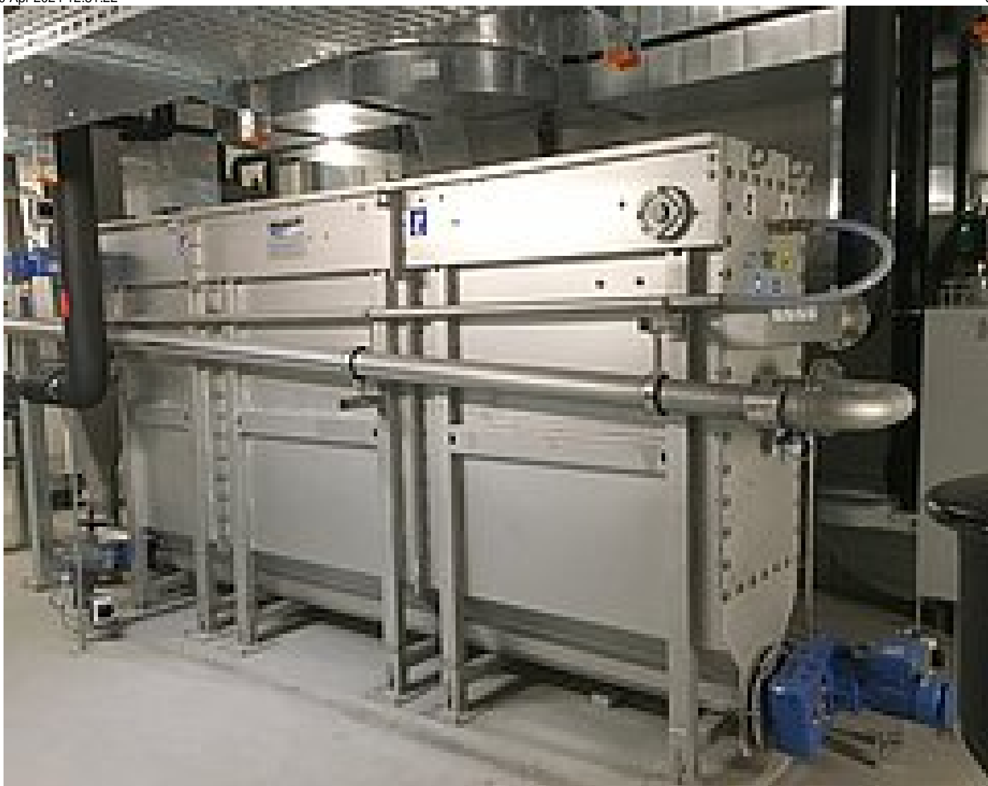
Fig. 3: HUBER Heat Exchanger RoWin in the technical equipment room of the Valsana hotel
