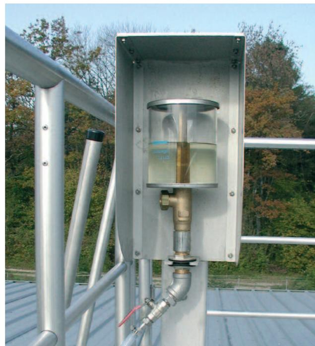
Leak control for VRM® bearing
