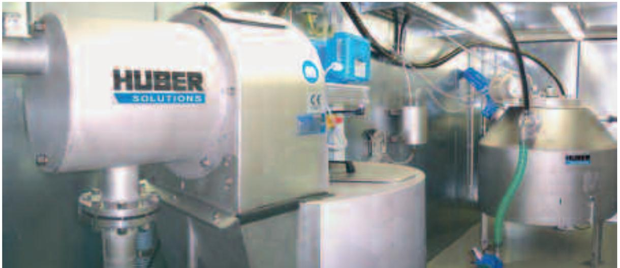
*Anaerobic reactor for the digestion of black or brown water*
