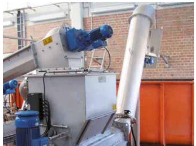
HUBER Screw Conveyor Ro8 T discharging screenings into a HUBER Wash Press WAP® SL.
