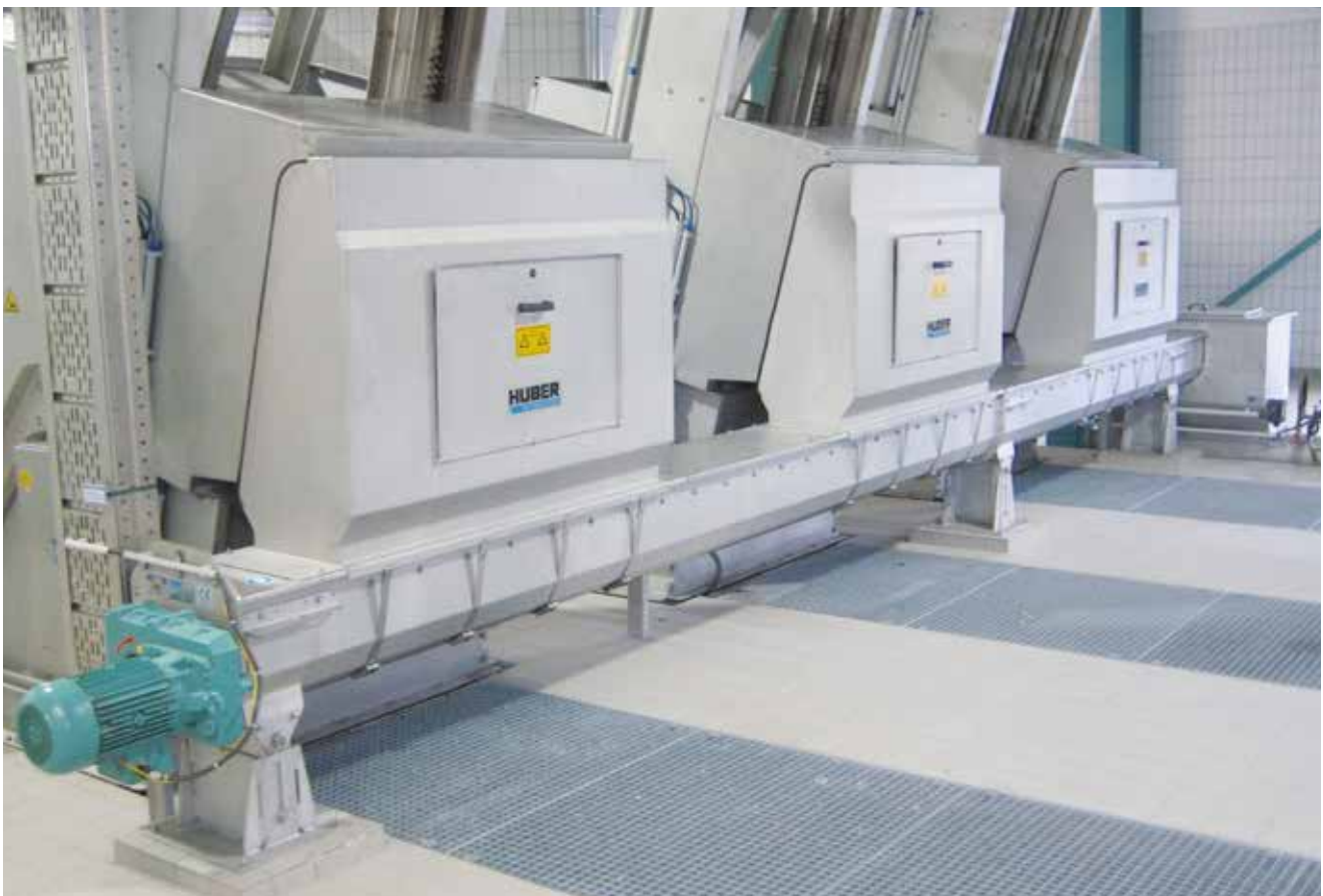
Three screens discharging screenings into a HUBER Screw Conveyor Ro8 T.
