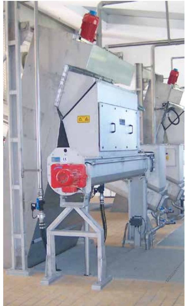
Side view of an enclosed HUBER Fine Screen STEP SCREEN® SSV for odour-free screenings discharge through the transfer chamber with screw conveyor.
