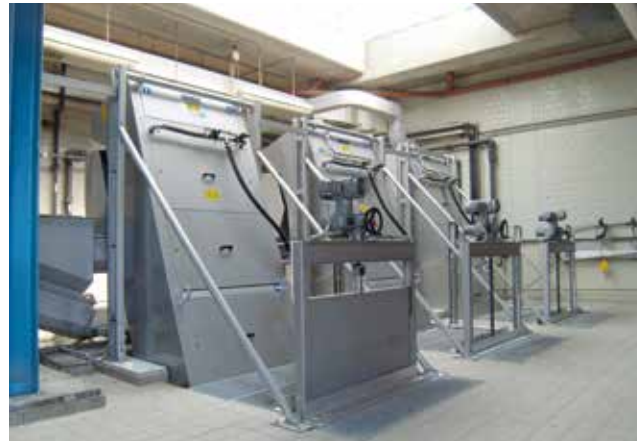
HUBER Fine Screen STEP SCREEN® SSV: 4300 mm long, 3 mm slot width, acid treated in a pickling bath for optimal corrosion protection.
