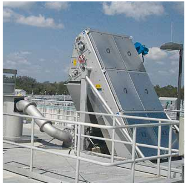
Fully enclosed, odour-free HUBER Belt Screen EscaMax® with easy to remove covers.
